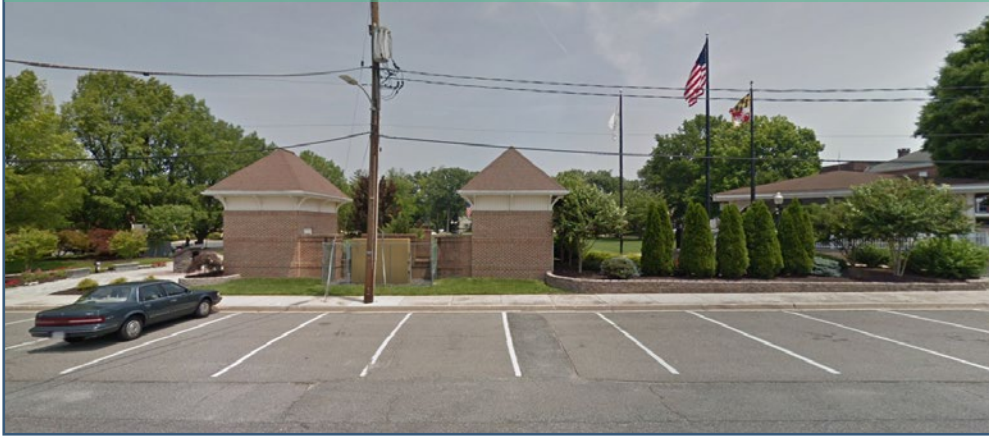
Visual and Physical Access at the Southern Edge is Blocked
