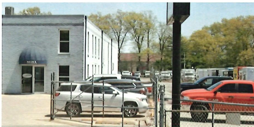
Looking East down south access lane to rear of the property
