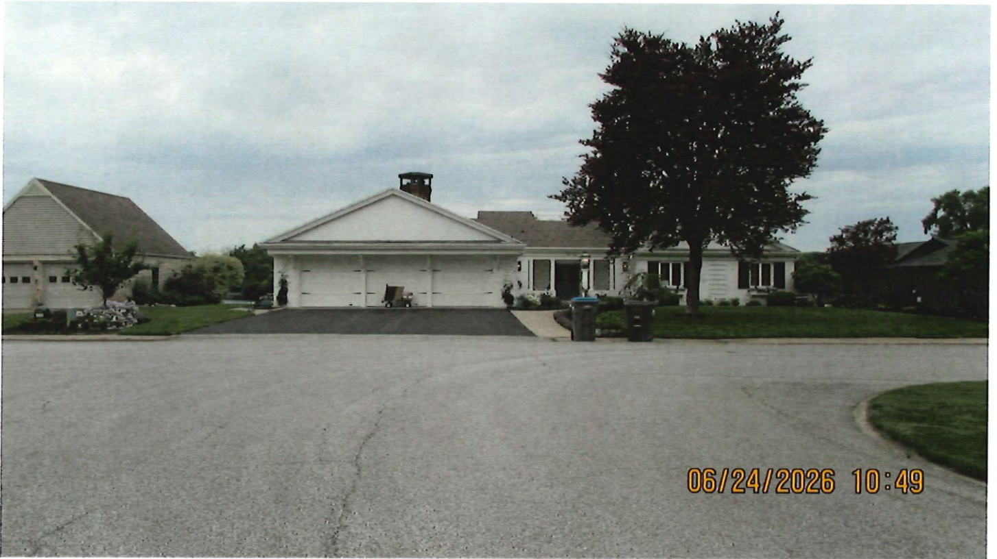
Looking North from Melrose Manor at petitioner's house
