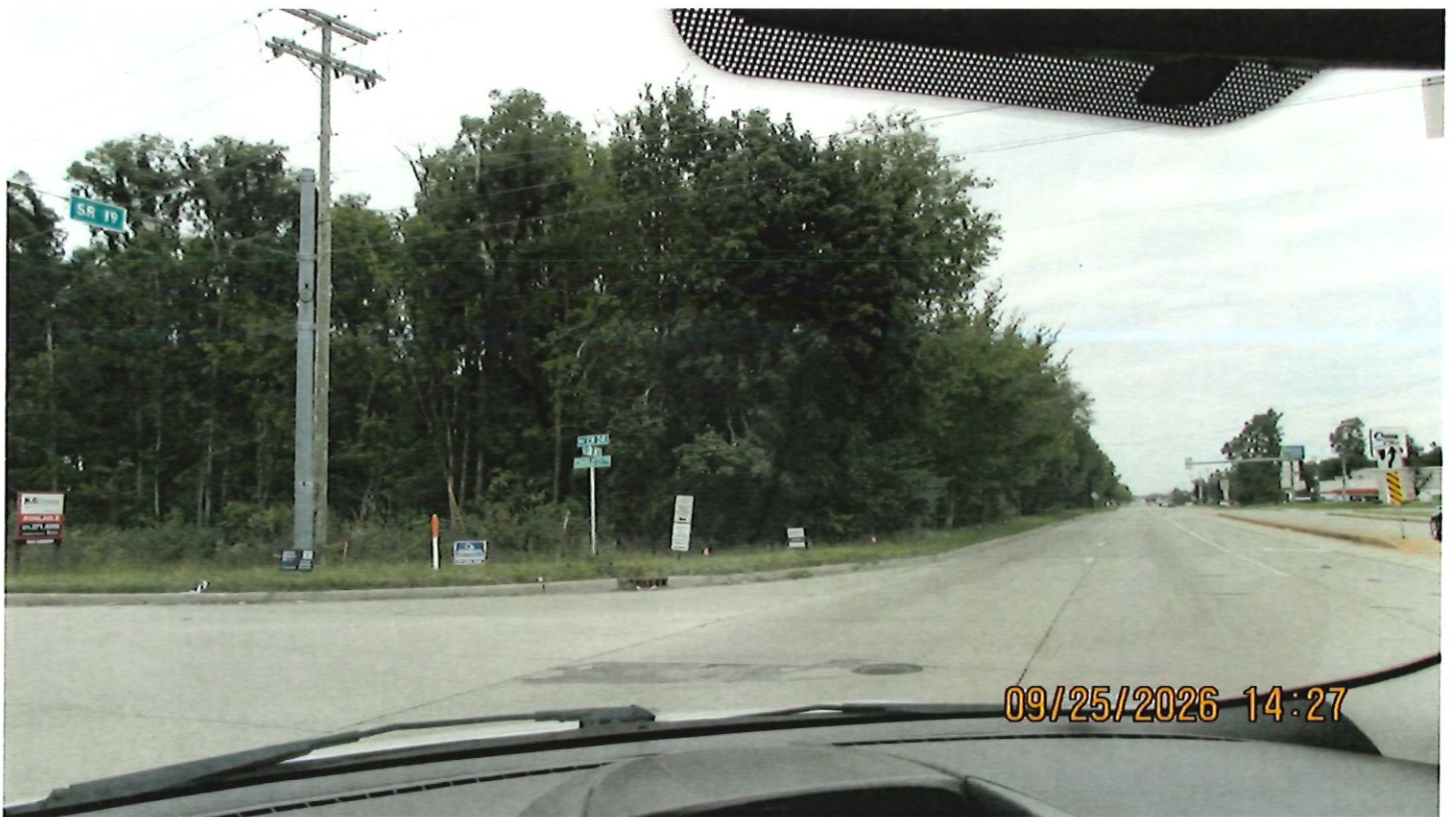
Site visit – looking NW from Charlotte & South Nappanee Street at proposed gas station site
