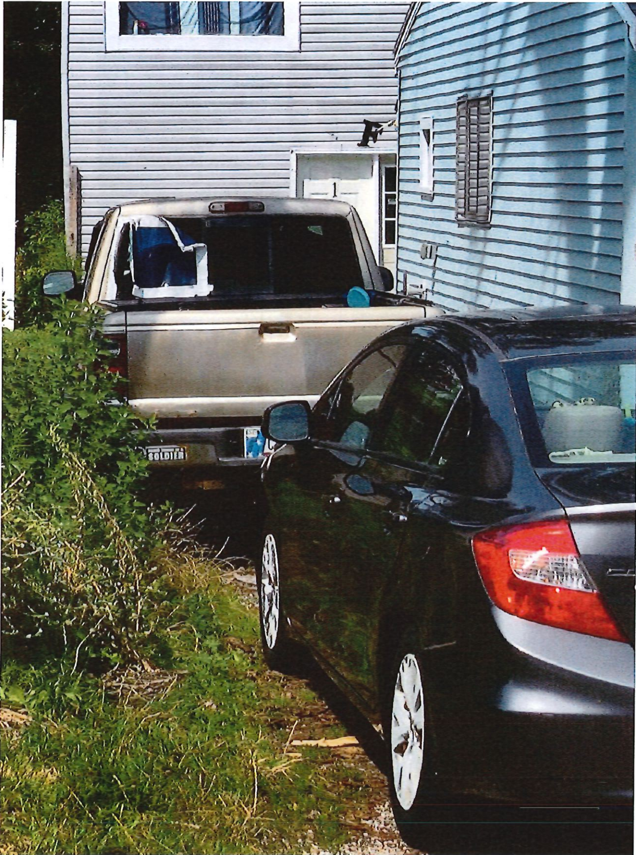
Below: Looking West at ADU in rear yard – close up
