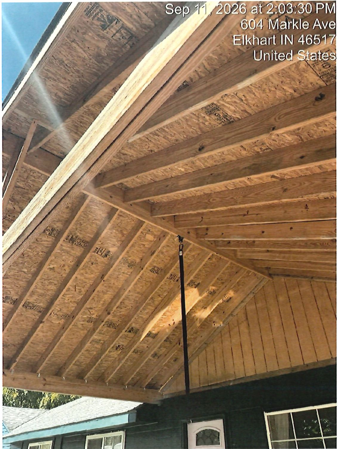
Site visit – viewing rafters standing outside the porch
