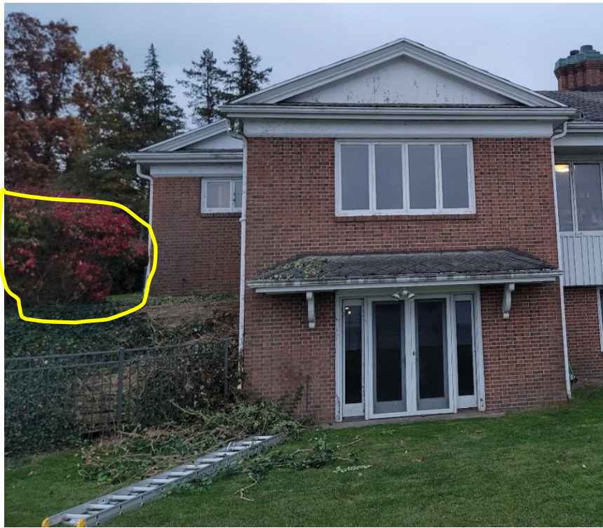
Picture taken before hedge removal showing height of more than 6 feet.
