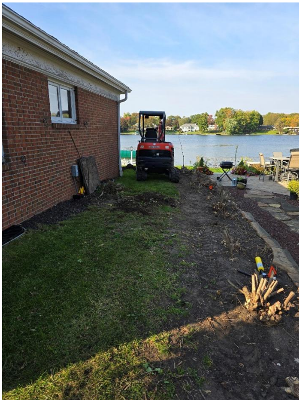
Temporary removal of privacy hedge and A/C unit in anticipation/preparation of construction.
