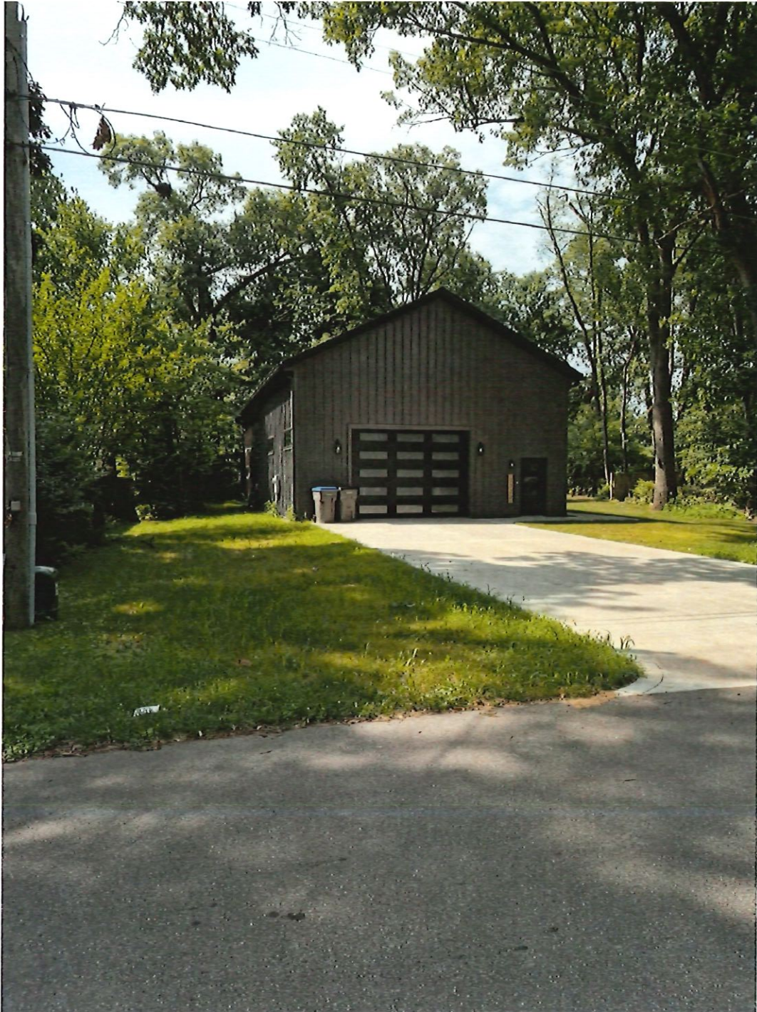
Below: Looking South at front of house
