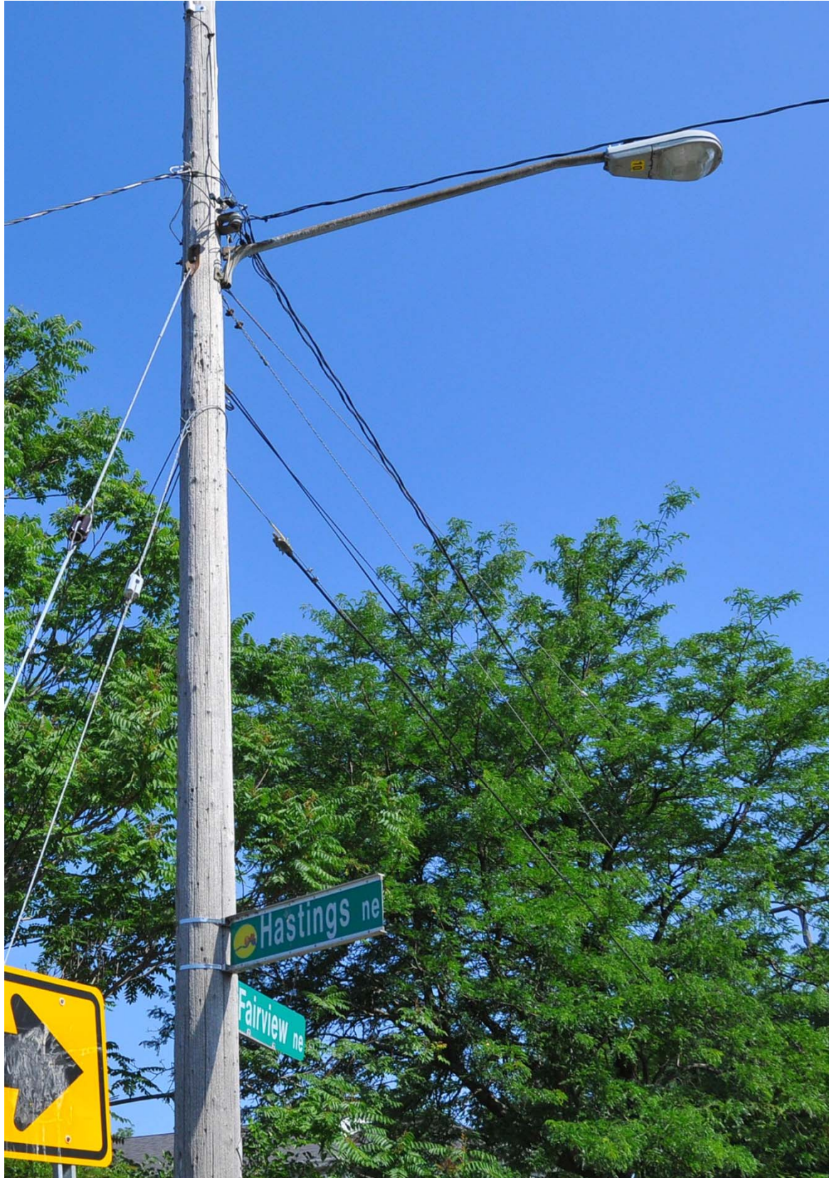
P1 Wood Pole with Cobra Head Luminaire
