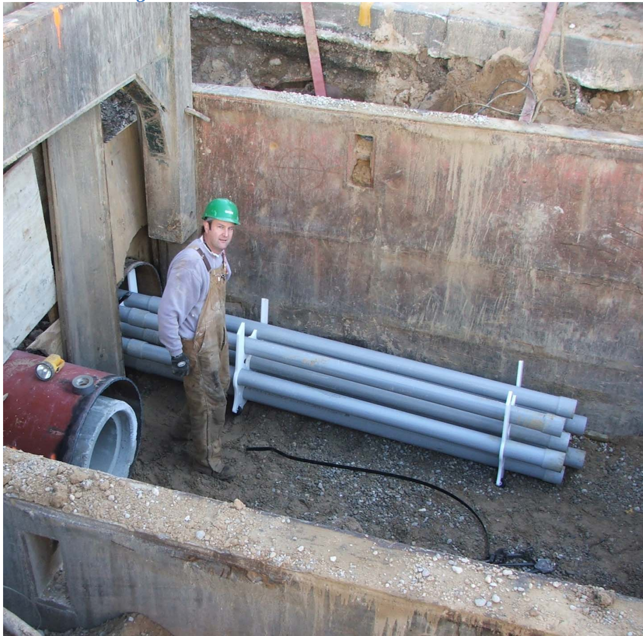
P5 Duct alongside Storm Sewer under US131
