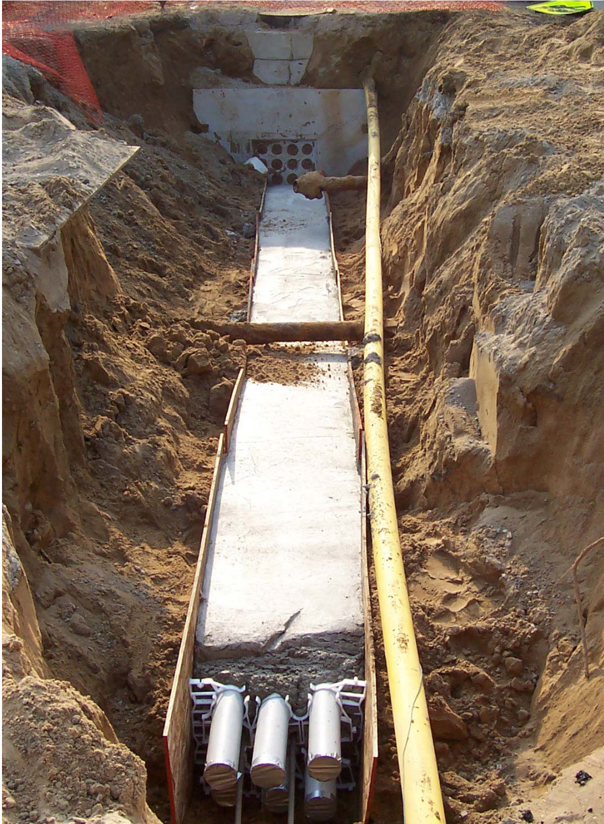
P6 Duct Installation in Wealthy Street
