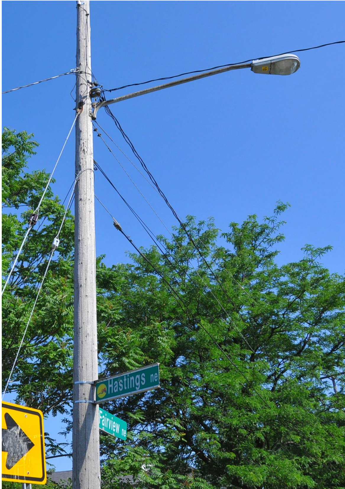
P1 Wood Pole with Cobra Head Luminaire
