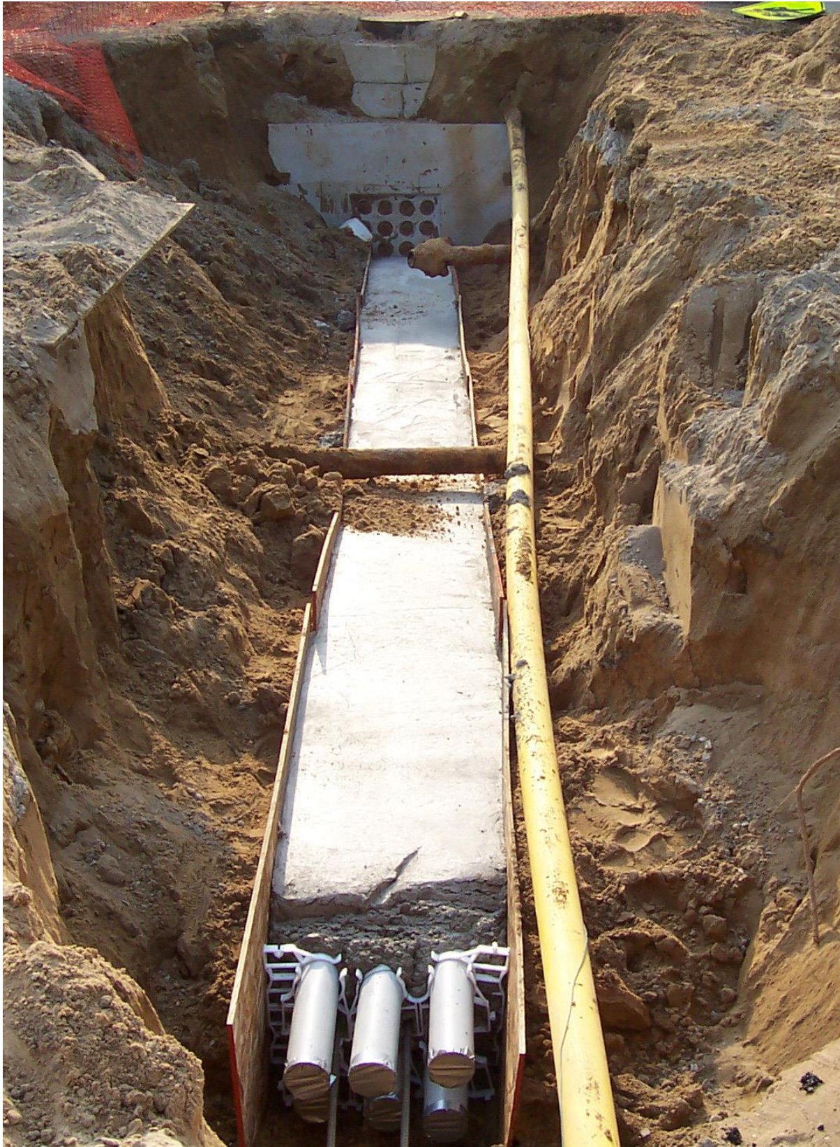
P6 Duct Installation in Wealthy Street
