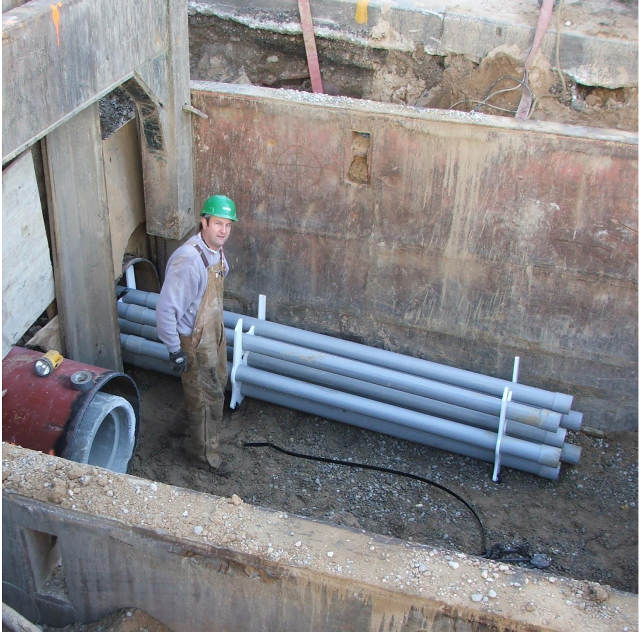
P5 Duct alongside Storm Sewer under US131
