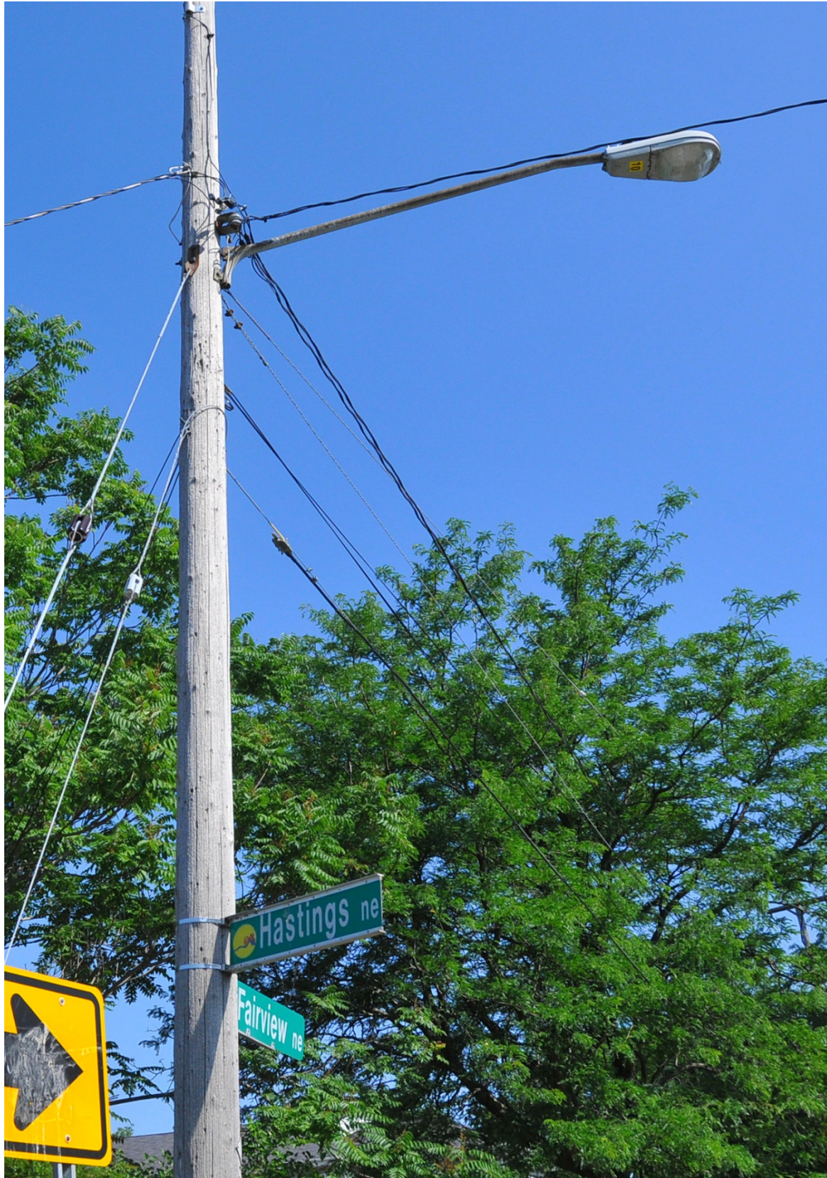
P1 Wood Pole with Cobra Head Luminaire
