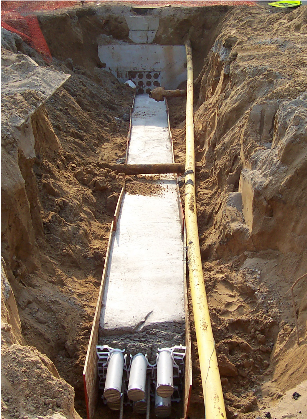
P6 Duct Installation in Wealthy Street
