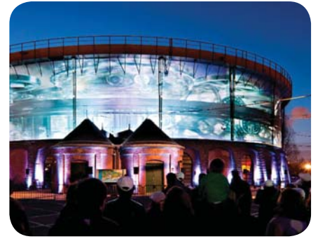
④ Repurposed water tank
