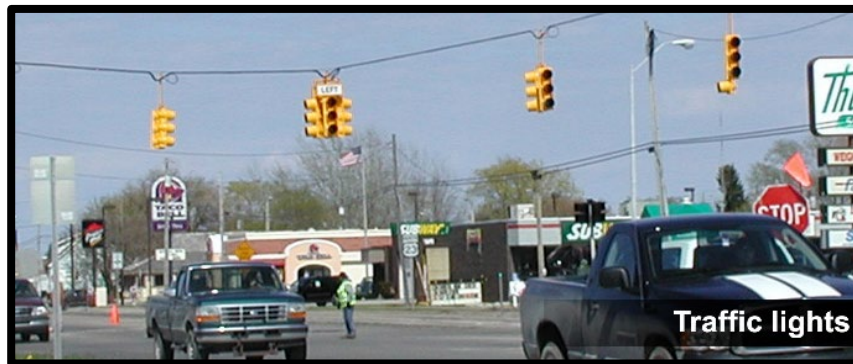
Figure D-1: Example of traffic signals
