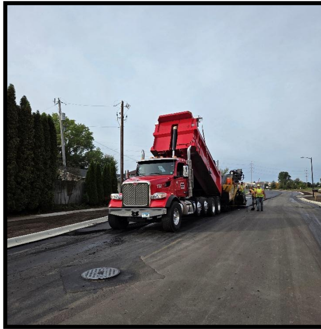
Paving the final lift on Pleasant Drive
