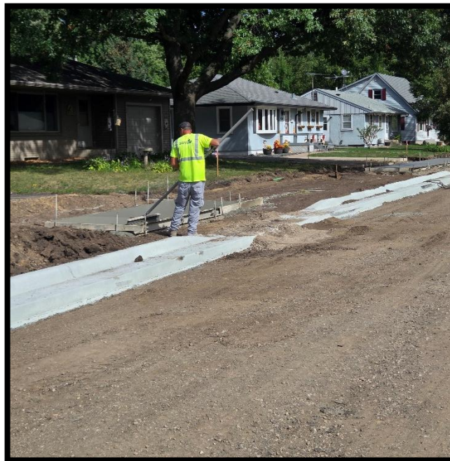
Concrete curb and driveway construction
