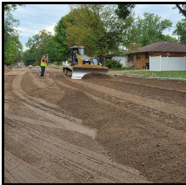
Excavation and preparation of road base
