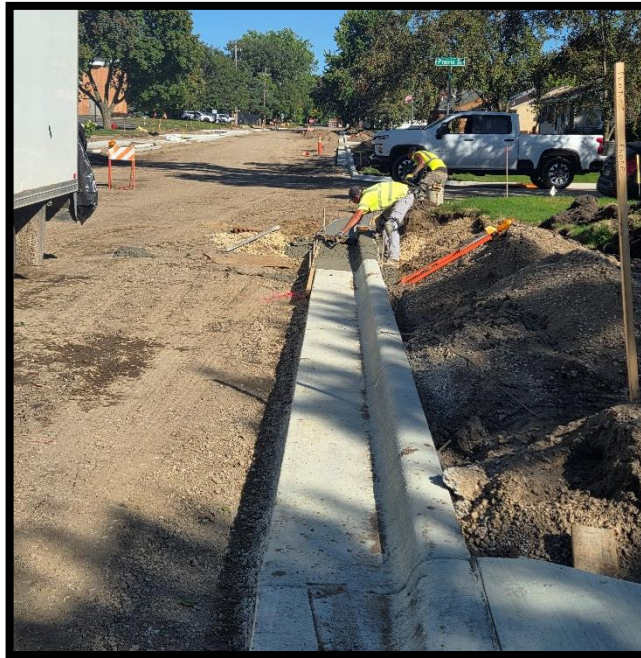
Concrete curb and driveway construction
