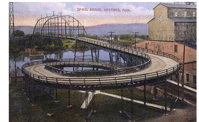
Obligatory image of the Spiral Bridge.
