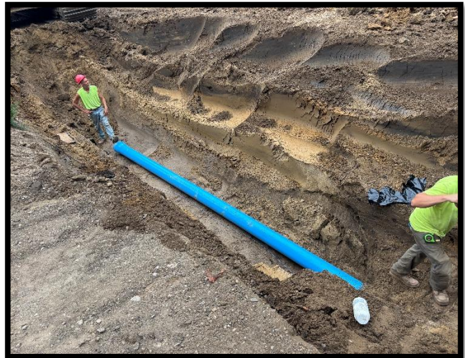
Watermain improvements on 4 th Street
