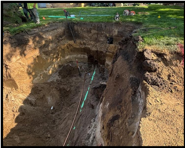
Sanitary sewer and watermain service improvements
