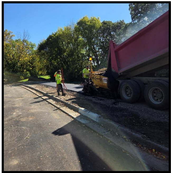
Paving of Lions Park Trail
