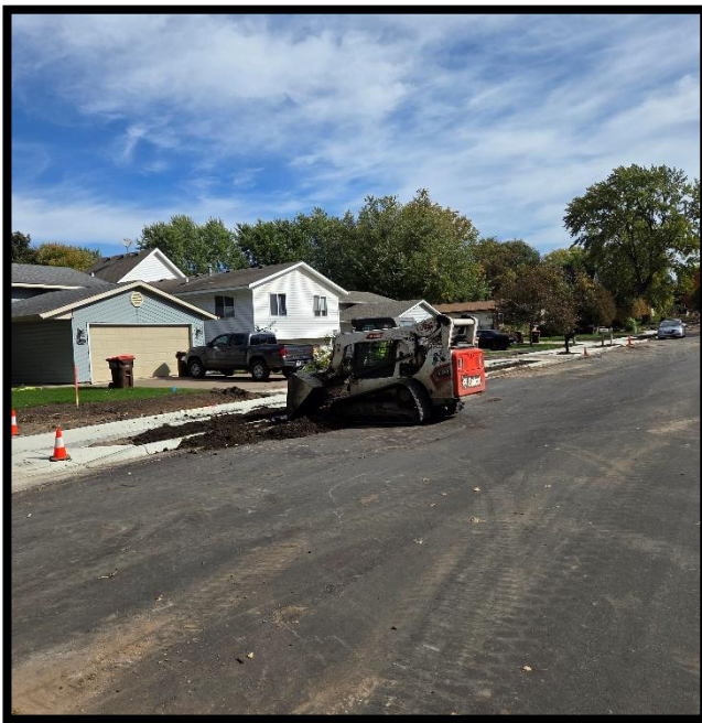
Boulevard grading along 4 th Street
