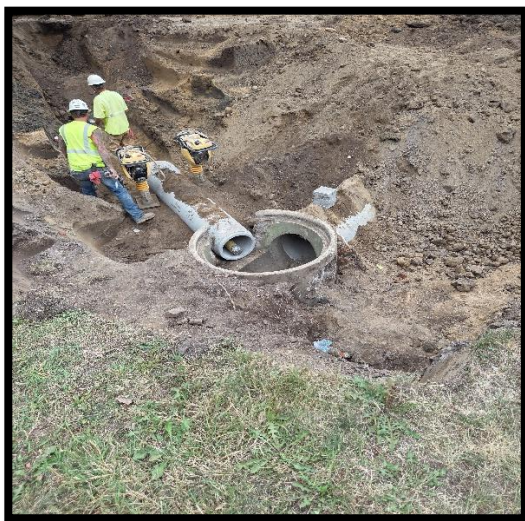
Storm sewer improvements
