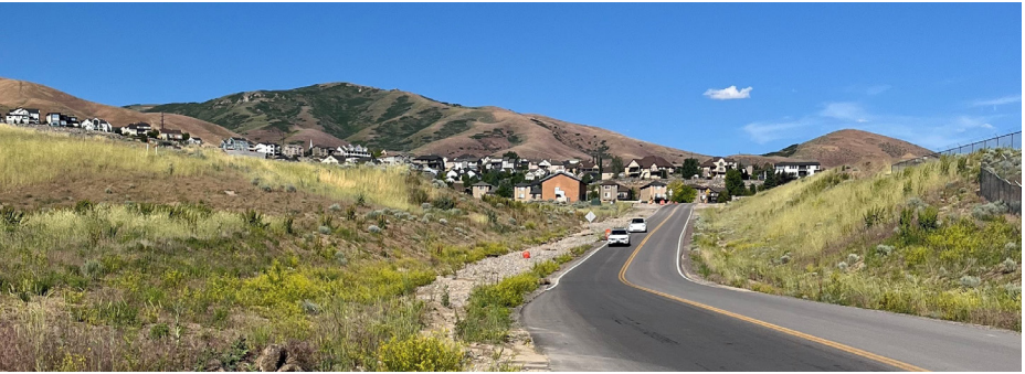
TRAVERSE MOUNTAIN BLVD
