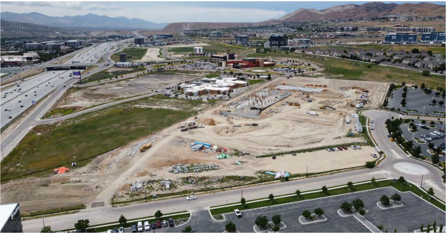
The Sanctuary housing development under construction, June 2023.
