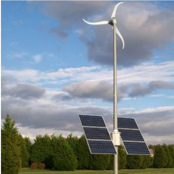
Figure 2. Hybrid wind and solar energy facility
