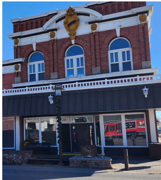
Reduced setbacks, distinct building base, large storefront windows
