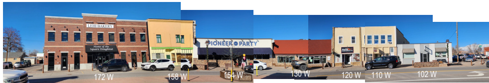
ELEVATION B - NORTH SIDE OF MAIN STREET BETWEEN 100 W STREET AND 200 W STREET
