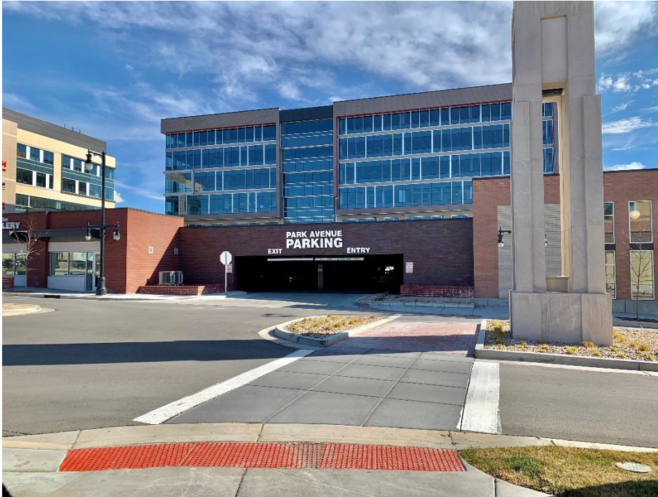
Figure 14. Pedestrian refuge within a central median.
