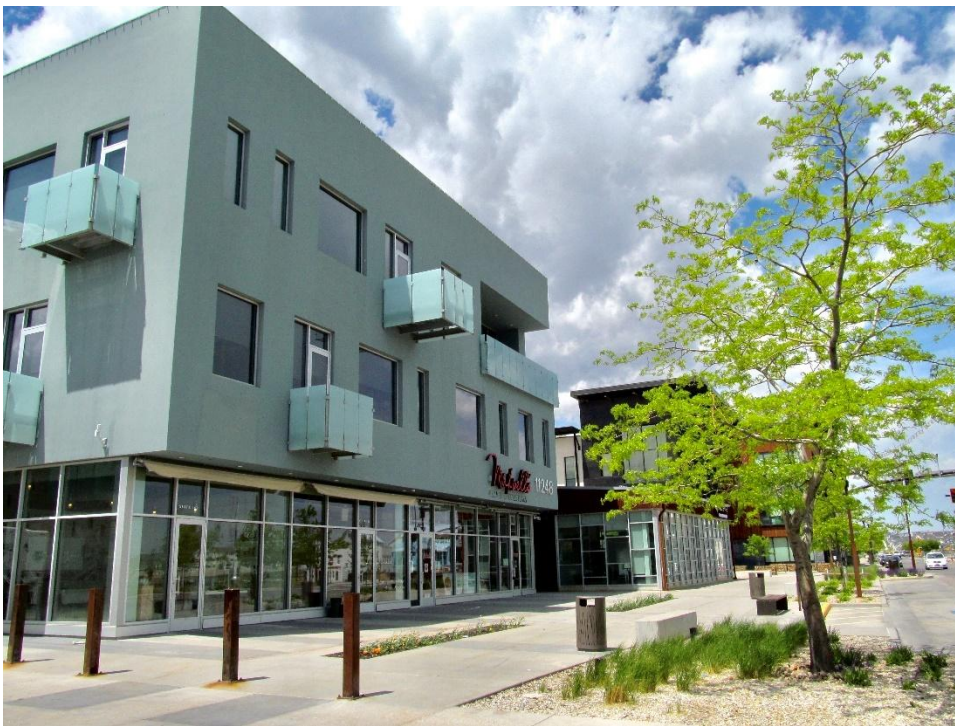
Figure 5. Retail building with clear windows on the ground floor exceeding 50% of the front façade.
