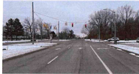
Southbound Hagadorn Road at Hannah Boulevard
