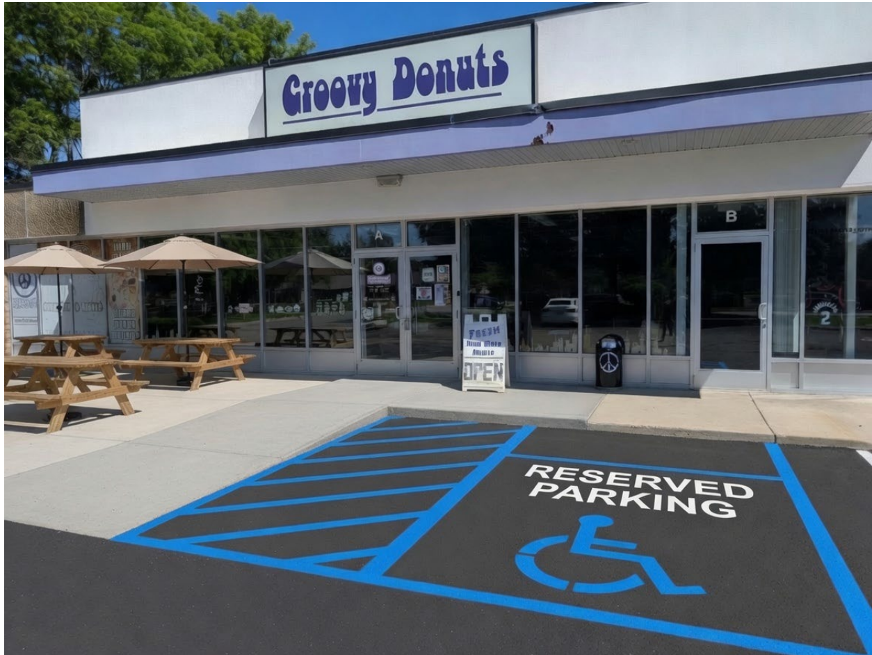
Completed project showing the new designated ADA-accessible parking space with diagonally striped access aisle directly in front of the storefront door, the new ADA-accessible customer patio with seating under umbrellas, and the resurfaced parking lot.
