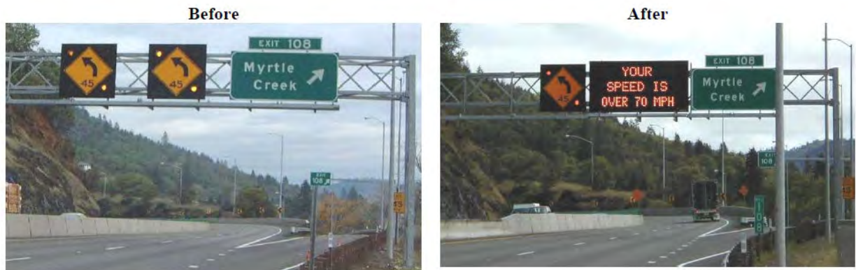
Figure 29. Curved section DSFS. (Before on left; after on right). (Bertini et al., 2006)
