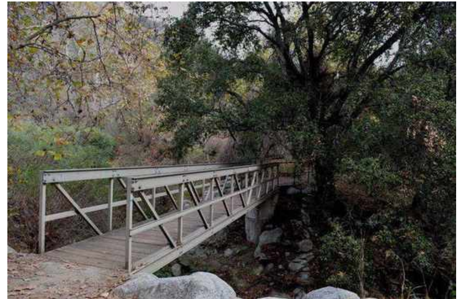
Existing footbridge during planning
