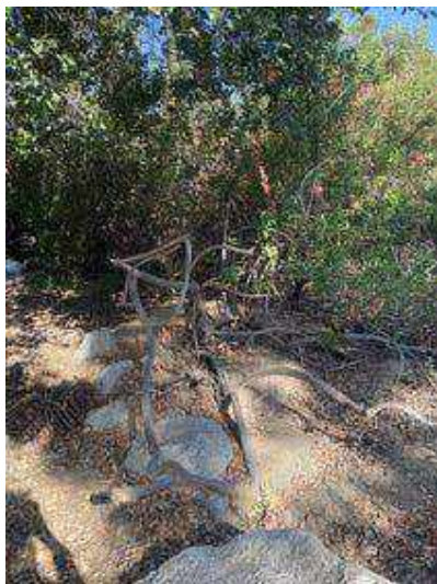
July 24, 2026: Work area before final vegetation treatment.
