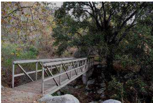
Bailey Canyon bridge area, existing footbridge condition documented during project planning.
