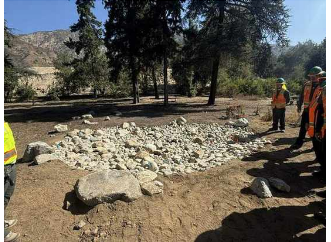
Second completed bioswale
