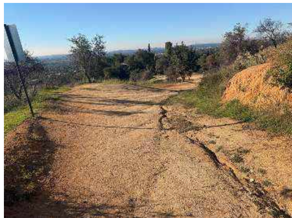
Mt. Wilson staging-area surface and drainage path, existing condition documented during project planning.
