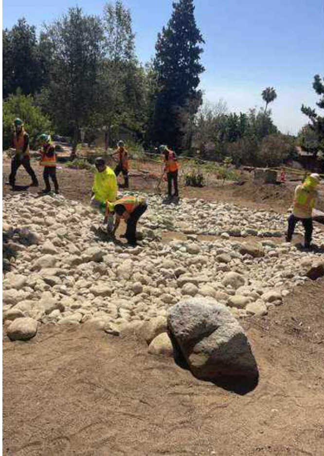
During rock placement
