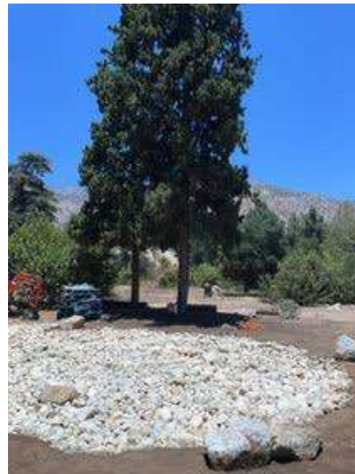
July 16, 2026: Constructed rock-lined drainage and stabilized work area.
