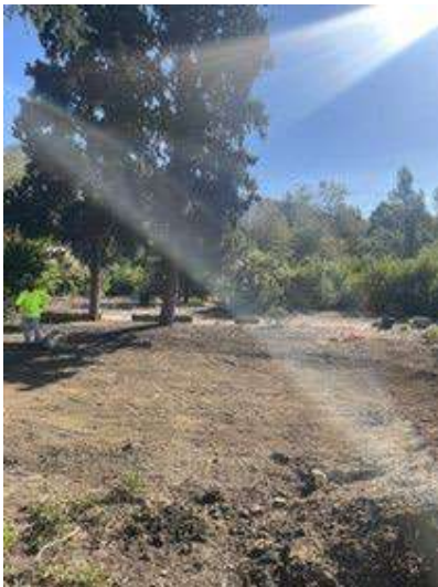
July 16, 2026: Rock placement and naturalized drainage construction in progress.
