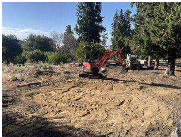
July 17, 2026: Site condition before drainage-area grading.
