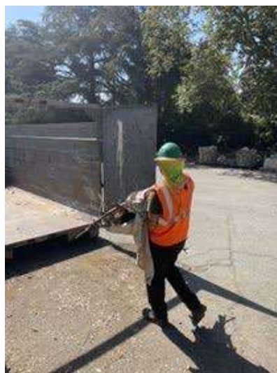
July 24, 2026: Crew removing final debris during project cleanup.
