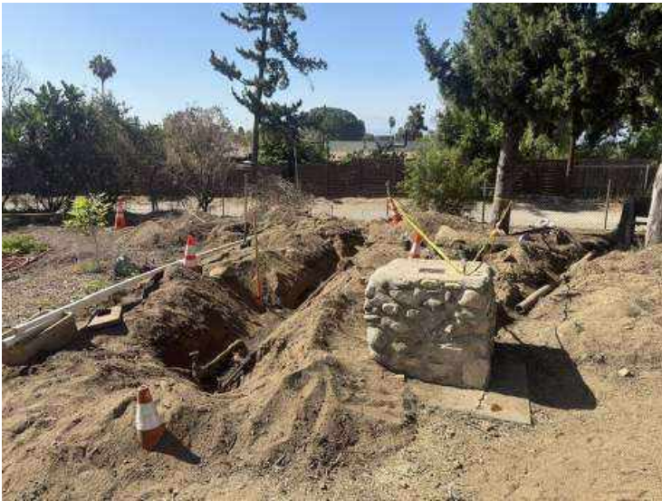
Irrigation installation
