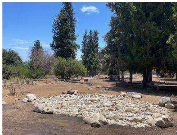
July 17, 2026: Same area after clearing and grading.
