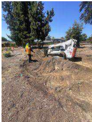
July 15, 2026: Work area during vegetation removal and site grading.
