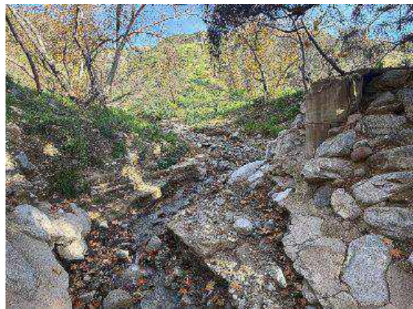
Bailey Canyon creek channel and bridge abutment area, existing condition documented during project planning.
